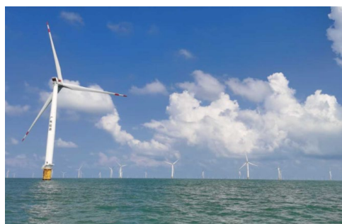
Offshore Wind Turbine Foundation Inspection
